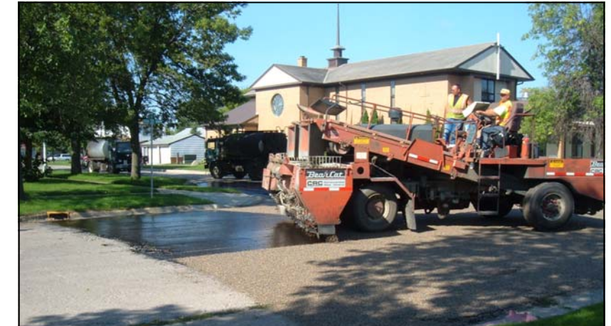
The crew from Astech applies the seal coat near First Lutheran Church on 5th Street NW.
