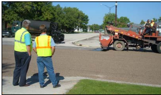
Above: Brad Bail and Steve Emery watch the application of a seal coat on the corner of Central Avenue and 6th St. NW. Right: Shawn Muhle inspects the seal coat project. Far right above: Steve Emery presents an aerial photo of the City of Badger to Clerk-Treasurer Pam Monsrud in honor of the community's centennial celebration. Far right below: Tom Stenseth checks out a low spot in the curb and gutter in EGF, which will be corrected during the mill and overlay application.
