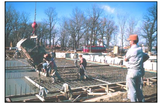
Construction of the East Grand Forks Water Treatment Plant in 1958.
